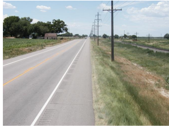
Figure S-6. Example of Inadequate Clear Zone along US 50
